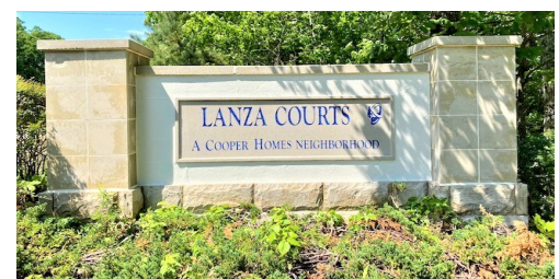
Lanza Courts sign—repaired and repainted.
