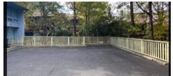
Castellon Courts—new railing installed for safety purposes.
