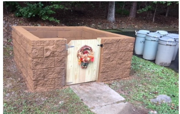
Newly Constructed Trash Corrals in Several Courts
